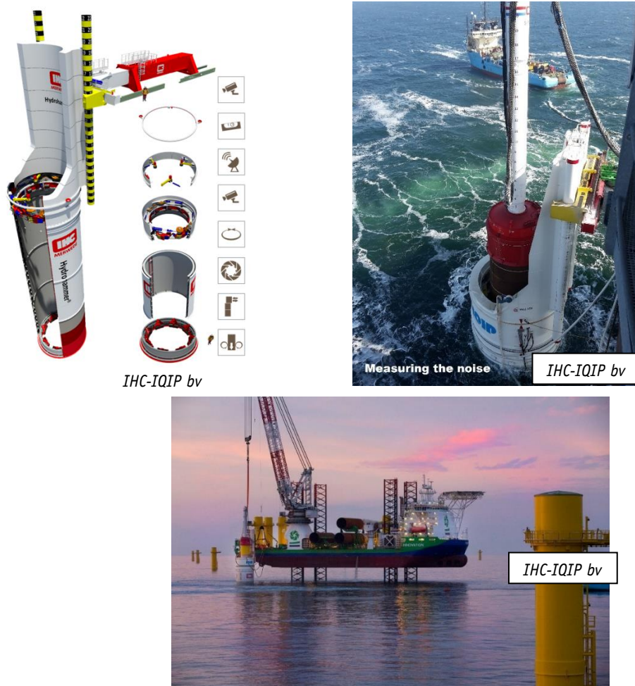
Figure 27: Noise Mitigation Screen of the company IHC IQIP bv. Top left: technical construction drawings of the double-walled steel tube incl. inside pile-sleeve; top right: IHC-NMS in offshore use (close-up); below: IHC-NMS in offshore use. (Source: IHC IQIP bv)
